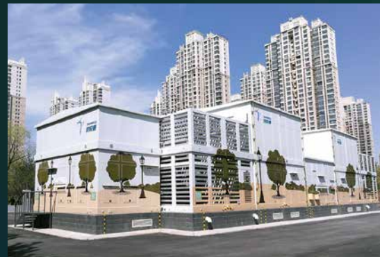
New construction of substation
