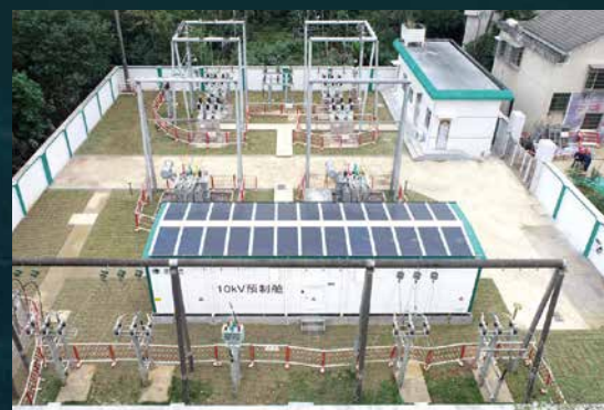
Substation technical renovation
