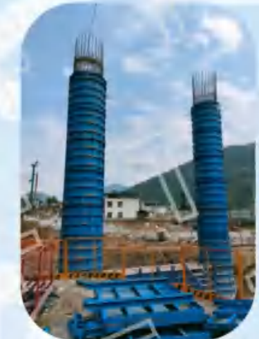
Pier Column Mold
