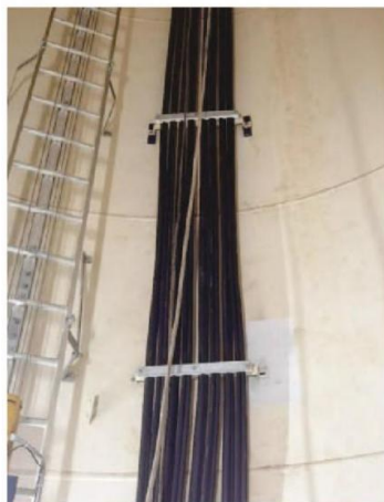
▲ repair broken nail fastener 磁吸补救射钉断裂点位
