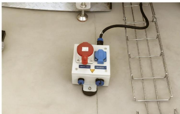
▲ socket fastened by magnets 磁吸插座
