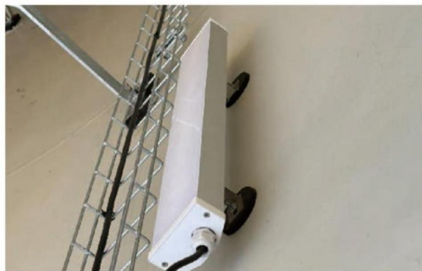
▲ Fastening light inside the wind tower 固定灯具
