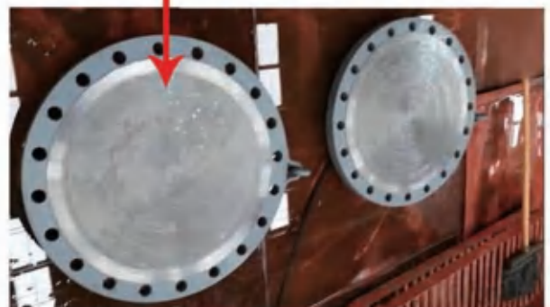
AFTER BEING REMOVED
