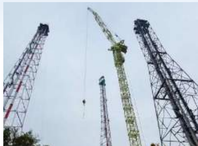
Petrochemical Torch Tower Overhaul
