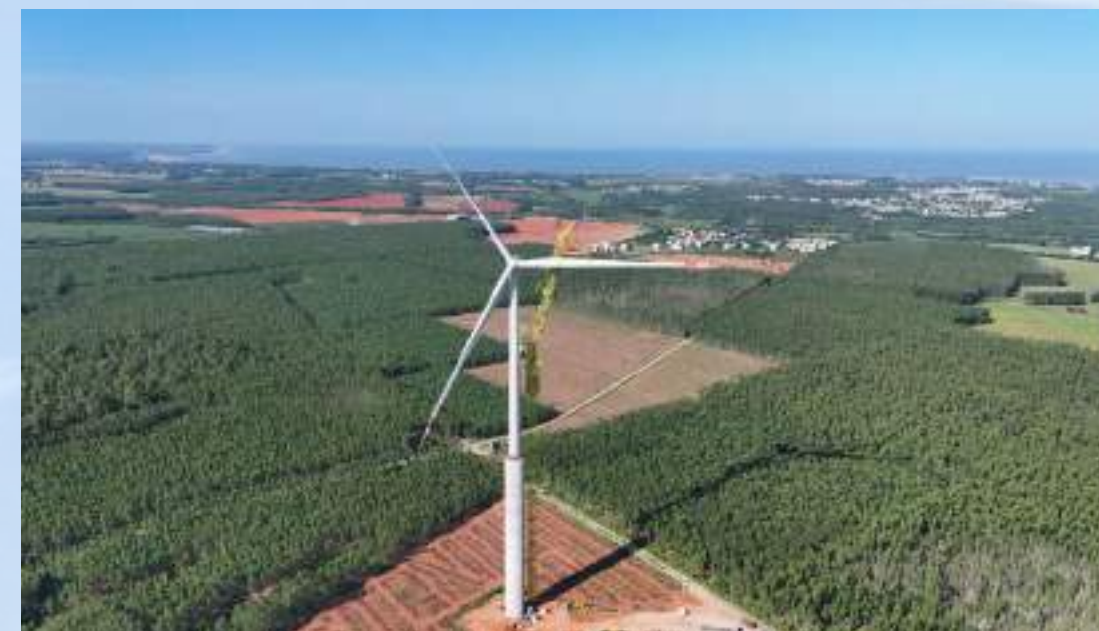
JLD 200t Luffing Jib Tower Crane for 5MW-185m Wind Power Hoisting
