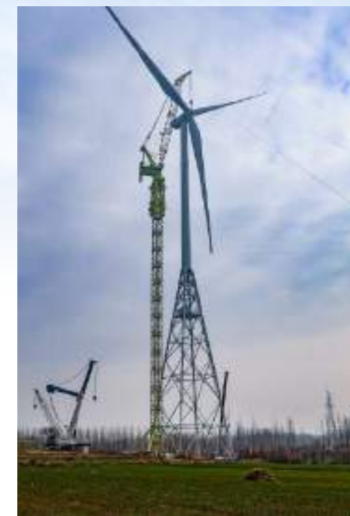
JLD 180t Luffing Jib Tower Crane for 4.5MW-160m Wind Power Hoisting
