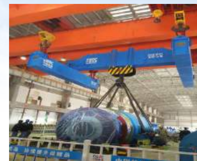
450t Special spreader for Generator stator
