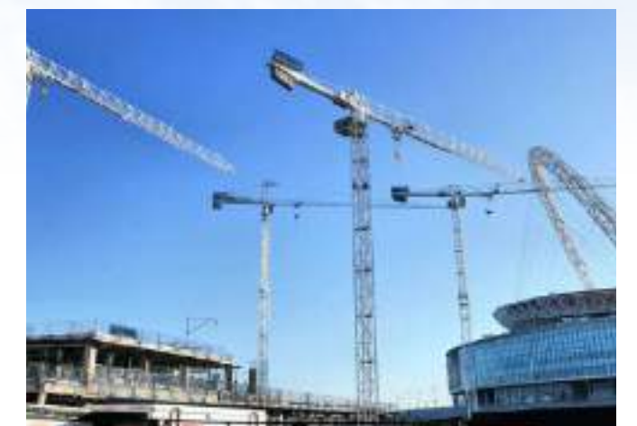
JLP Flat-Top Tower Crane for Stadium Construction
