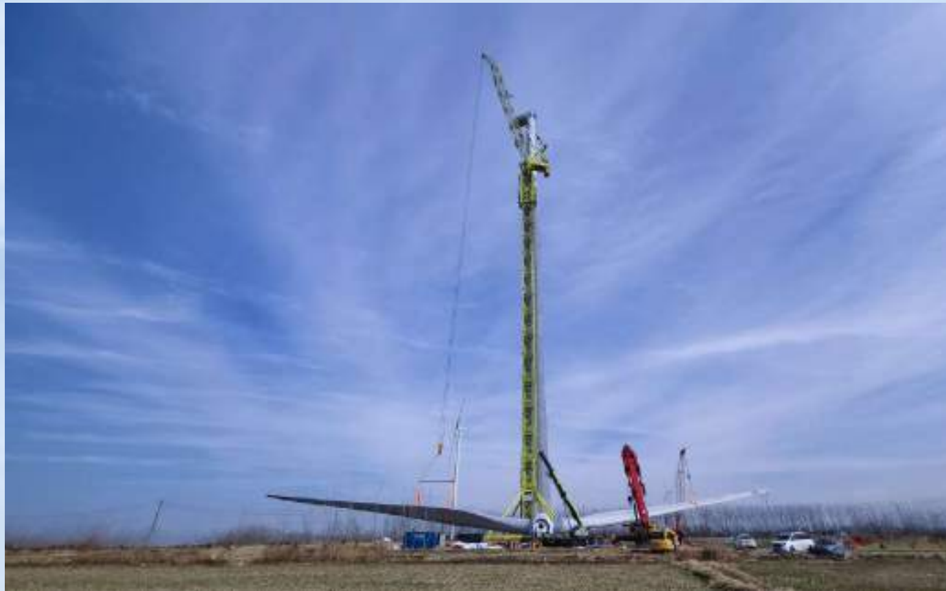
JLD 200t Luffing Jib Tower Crane for 5MW-180m Wind Power Hoisting
