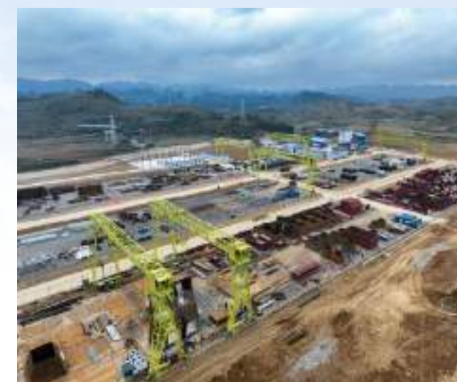
MDG Type Gantry Crane
