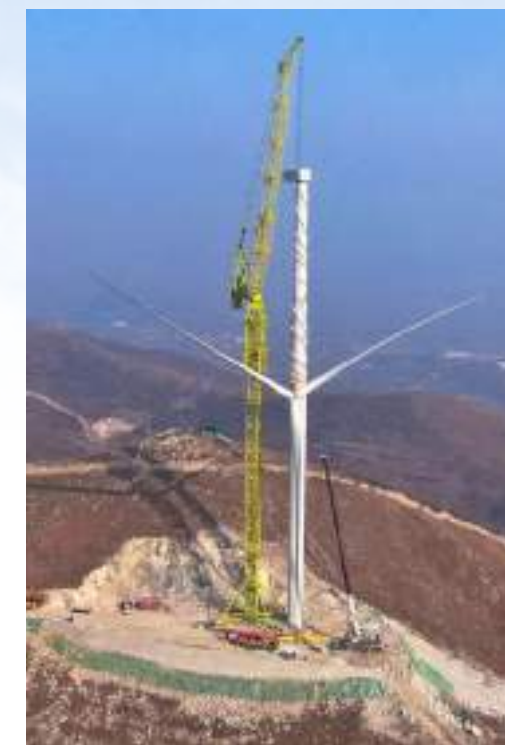
JLD 136t Luffing Jib Tower Crane for 2.2MW-130m Wind Power Hoisting
