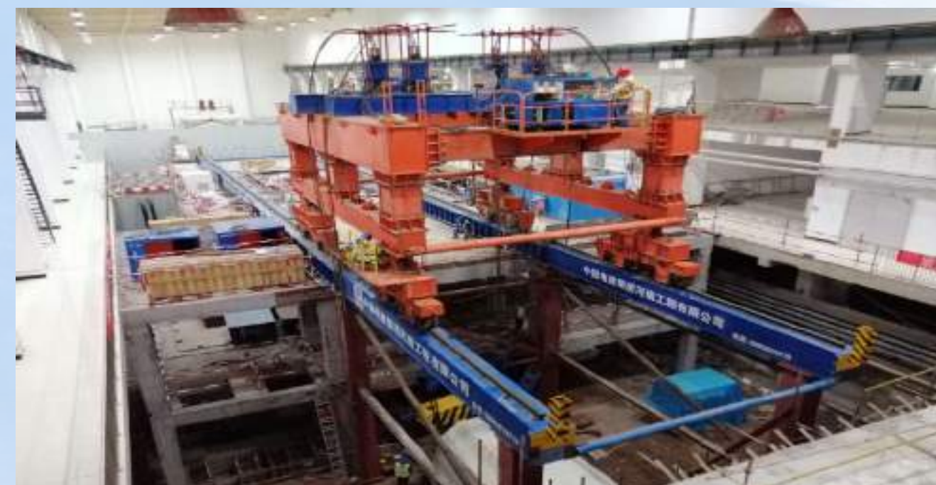
500t Special Designed Lifting tool for Generator Stator
