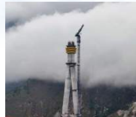
JLP Flat-Top Tower Crane for Bridge Construction
