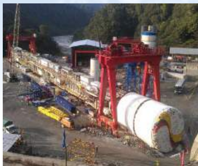
ME Type Gantry Crane for Subway Construction
