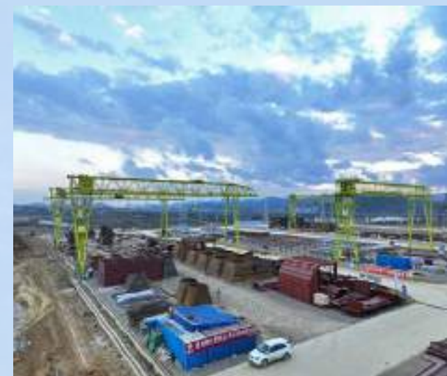
MDG Type Gantry Crane
