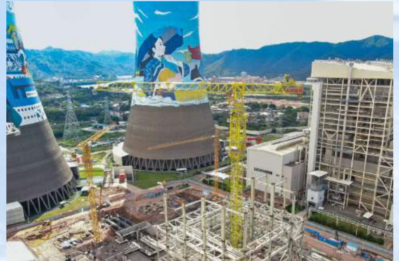
JLP 200t Flat-Top Tower Crane for Thermal Power Generating Unit Construction with the Large Chassis
