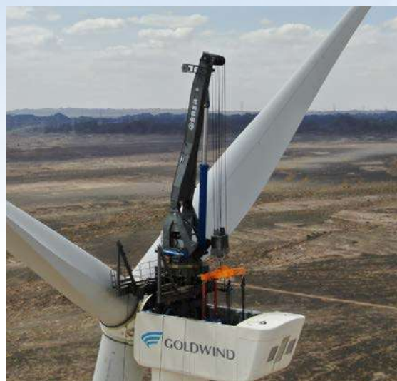
100t风机运维检修吊
