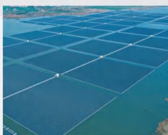
PLAIN PHOTOVOLTAIC POWER STATION
