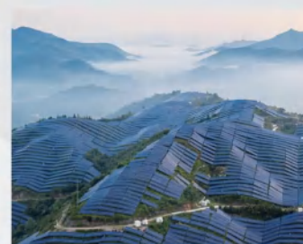
PLATEAU PHOTOVOLTAIC POWER STATION
