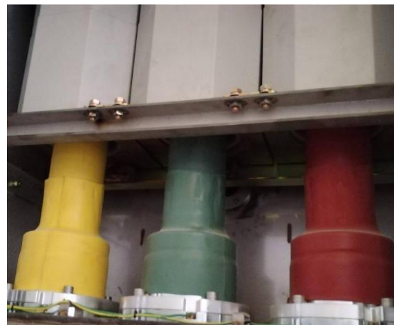
40.5kV/3150A Connection with SF 6 Gas-filled Switchgear
