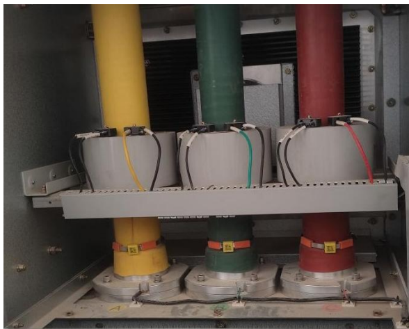
40.5kV/3150A SF 6 充气柜连接
