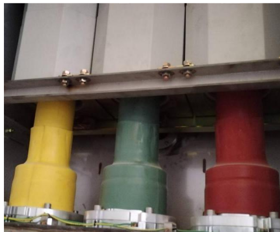
40.5kV/3150A SF 6 充气柜连接
