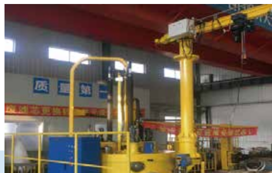
废滤芯更换转运单元 Filter replacement & transshipment unit
