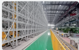
智能化立体仓库 Intelligent three-dimensional warehouse
