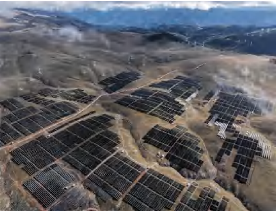
Figure: Aerial view of Xingchuan Empirical Photovoltaic Power Station.
