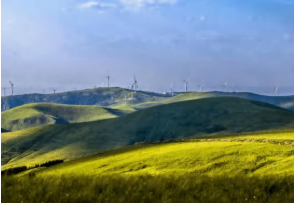
Figure: On-site of the Lan County Wind Power Project
