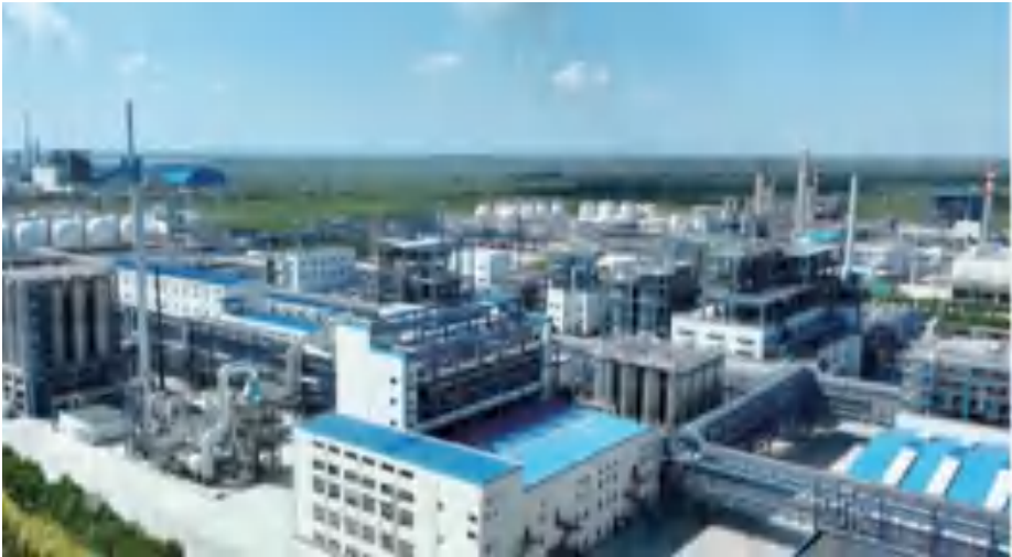
Figure: Lijin Refining & Chemical
