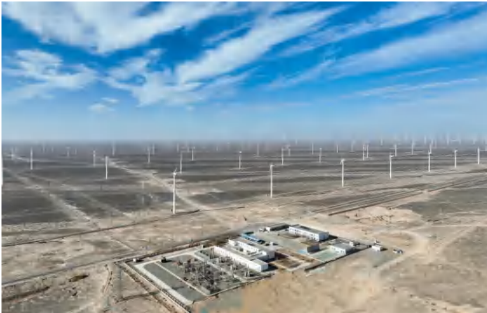
Figure: Aerial view of the project
