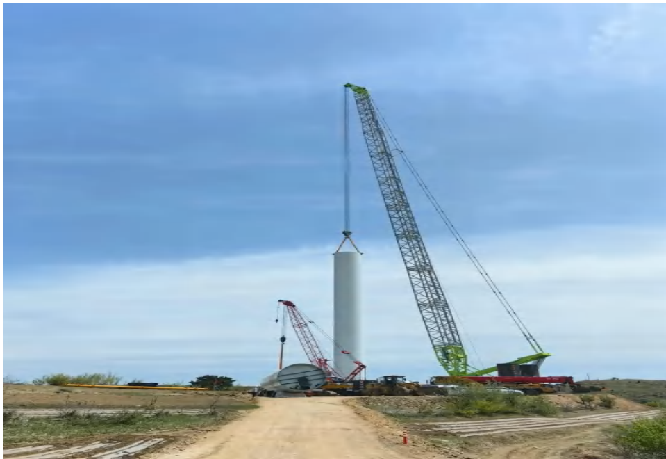
Figure: Project construction site.
