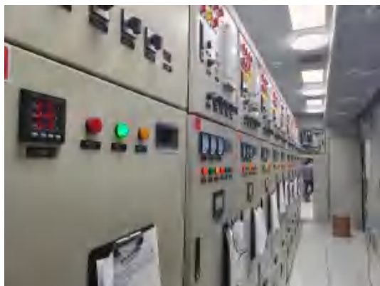
Ganzi Prefecture Project, Sichuan
