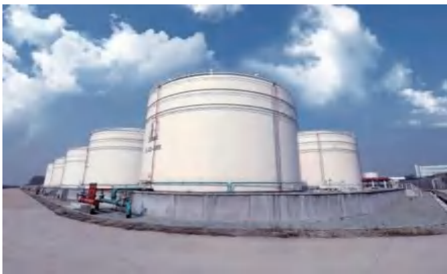
Figure: Sinochem Xingzhong Crude Oil Tank Area Phase 6 Expansion Project
