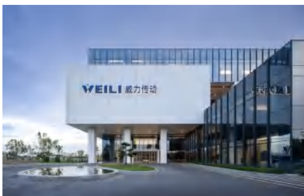
综合楼 Comprehensive Building
