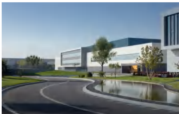
减速器厂区 Reducer factory area
