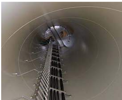
Mechanical Tower Internals (MTI)
