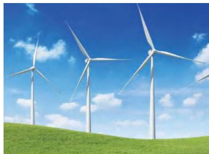
Wind power generation
